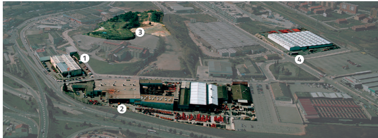
1. Headquarters 2. Assembly plant 3. Test, demonstration and training area 4. Warehouse for completed machines
